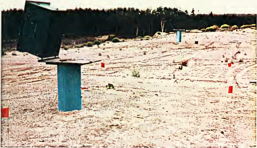
A 24: COMPLETED CONSTRUCTION, (BARRIE) SHOWING WELL COVERS
